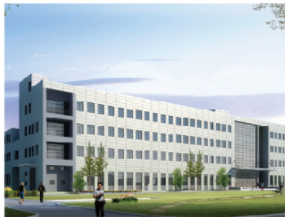
Beijing Zhongguancun Yongfeng Industrial Base Place: Beijing Area: 40000m 2 Panel Type: Steel cementitious panel
