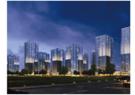
Yancheng Financial Center Place: Yancheng Area: 145700m 2 Panel Type: Steel cementitious panel
